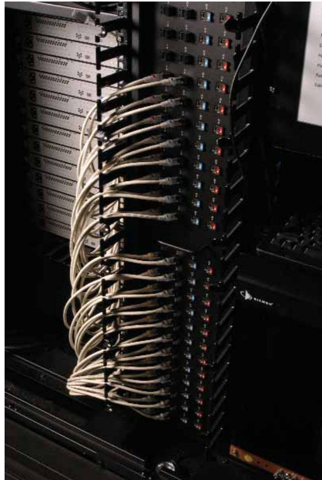
VersaPOD Zero-U Vertical Patch Panel
